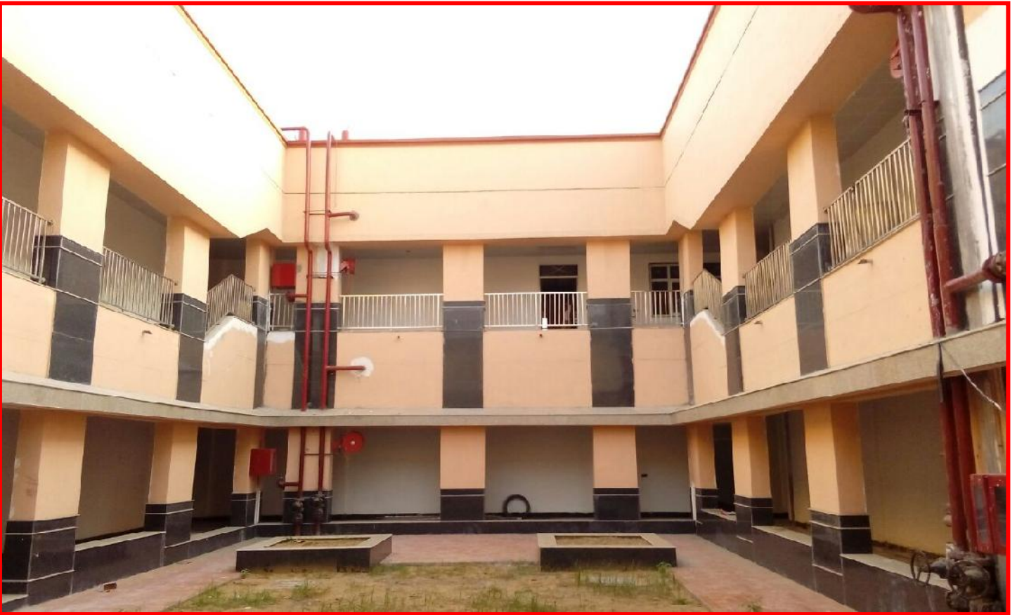
Training Infrastructure facilities at NSG Camp, Manesar
