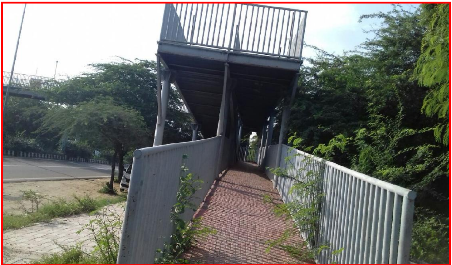
C/O Foot over bridge at Mehrauli Mahipalpur road New Delhi
