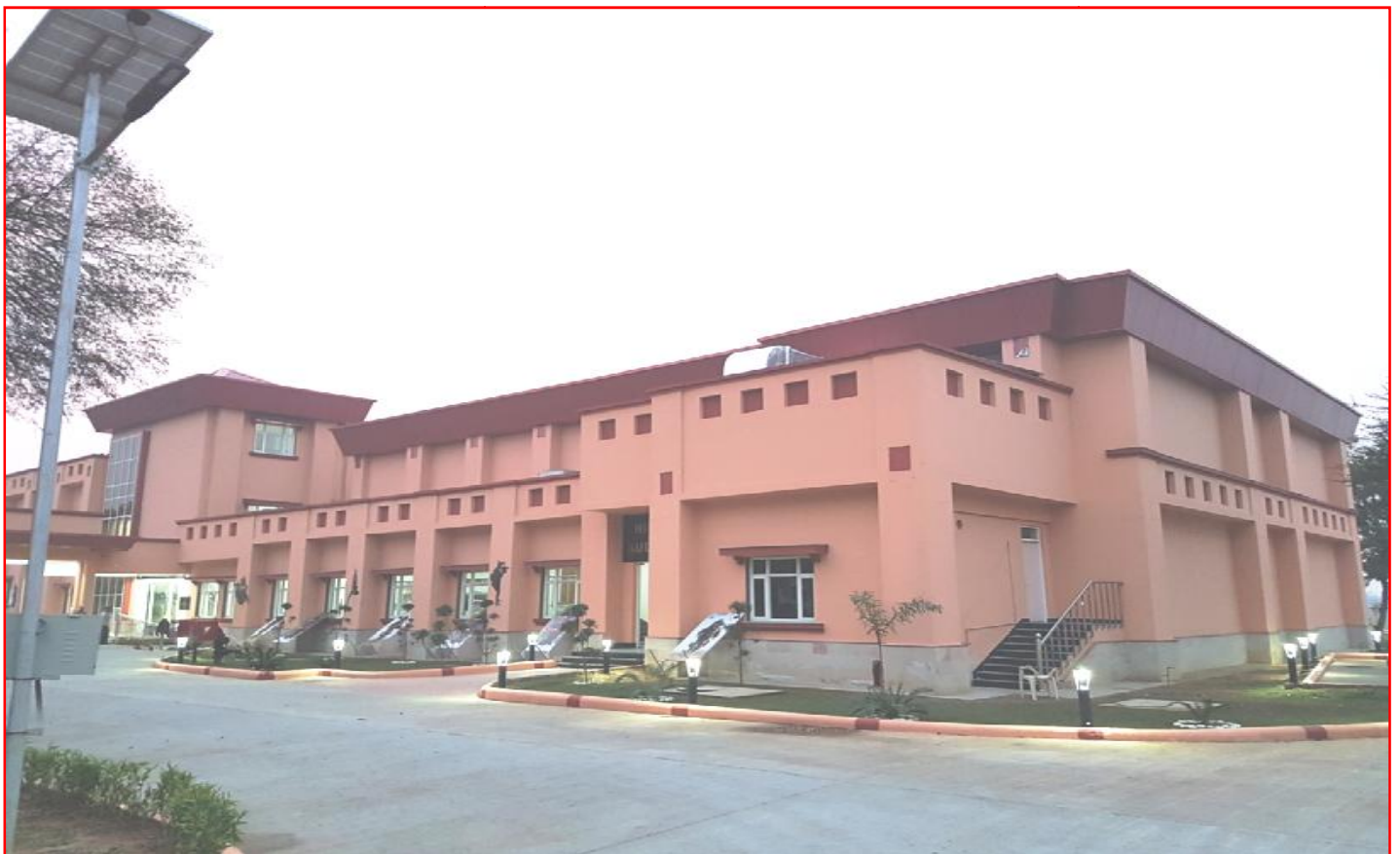
Training Infrastructure facilities/Auditorium at NSG Camp, Manesar
